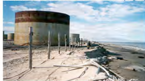
20 years ago these oil tanks were 60 m away from the coast of The Pechora Sea (Ogorogov, 2003)
